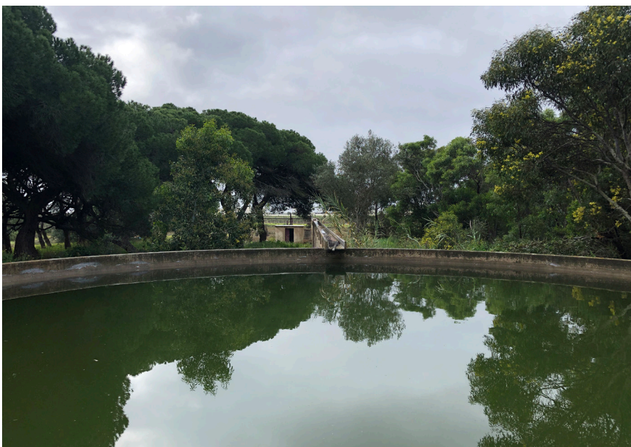
Hydraulic structures: tank, aqueduct and noria | photo Desidério Batista
