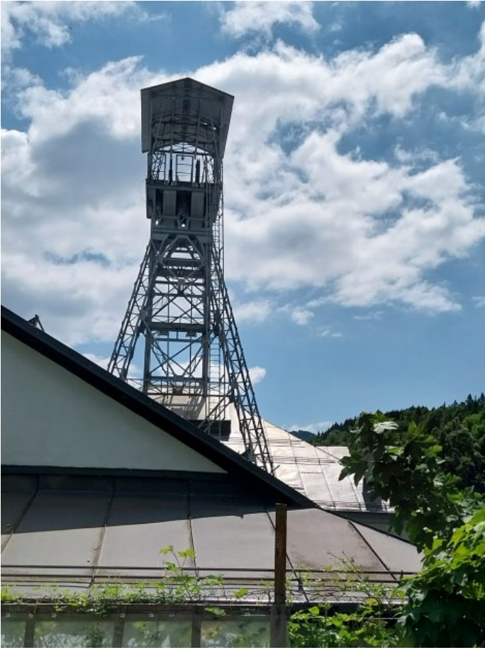
Mercury mine shaft
