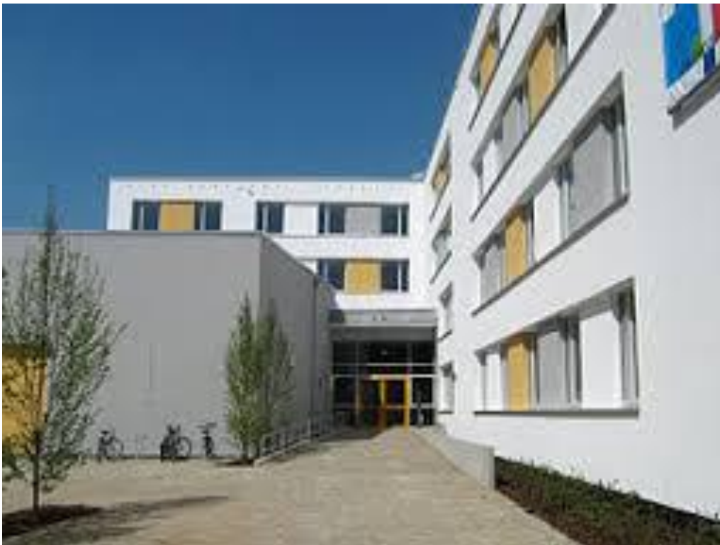
Figure: Frieda 23 building after restoration
