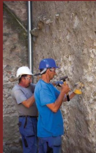
Exhausting removal of the cement mortar (Ižvolt and Smatanová 2014)
