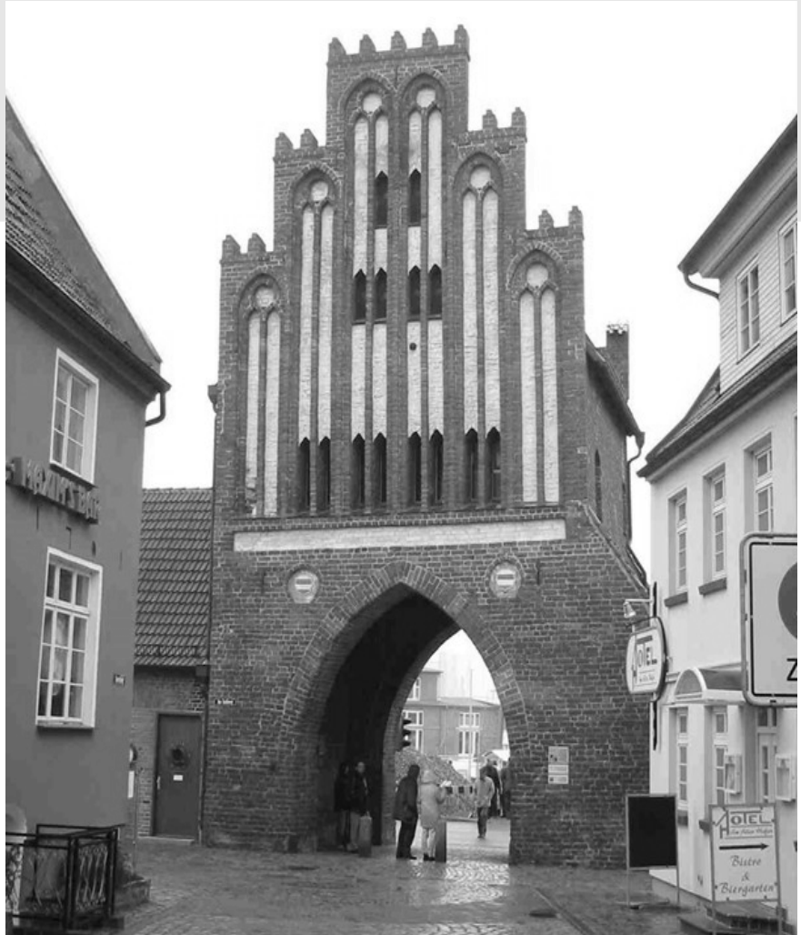
The water-tower of the hanseatic town Wismar was built during the Hanseatic period near the harbour. Today it is visualising the architecture of these days (Bernd Wollschläger, ALM MV).
